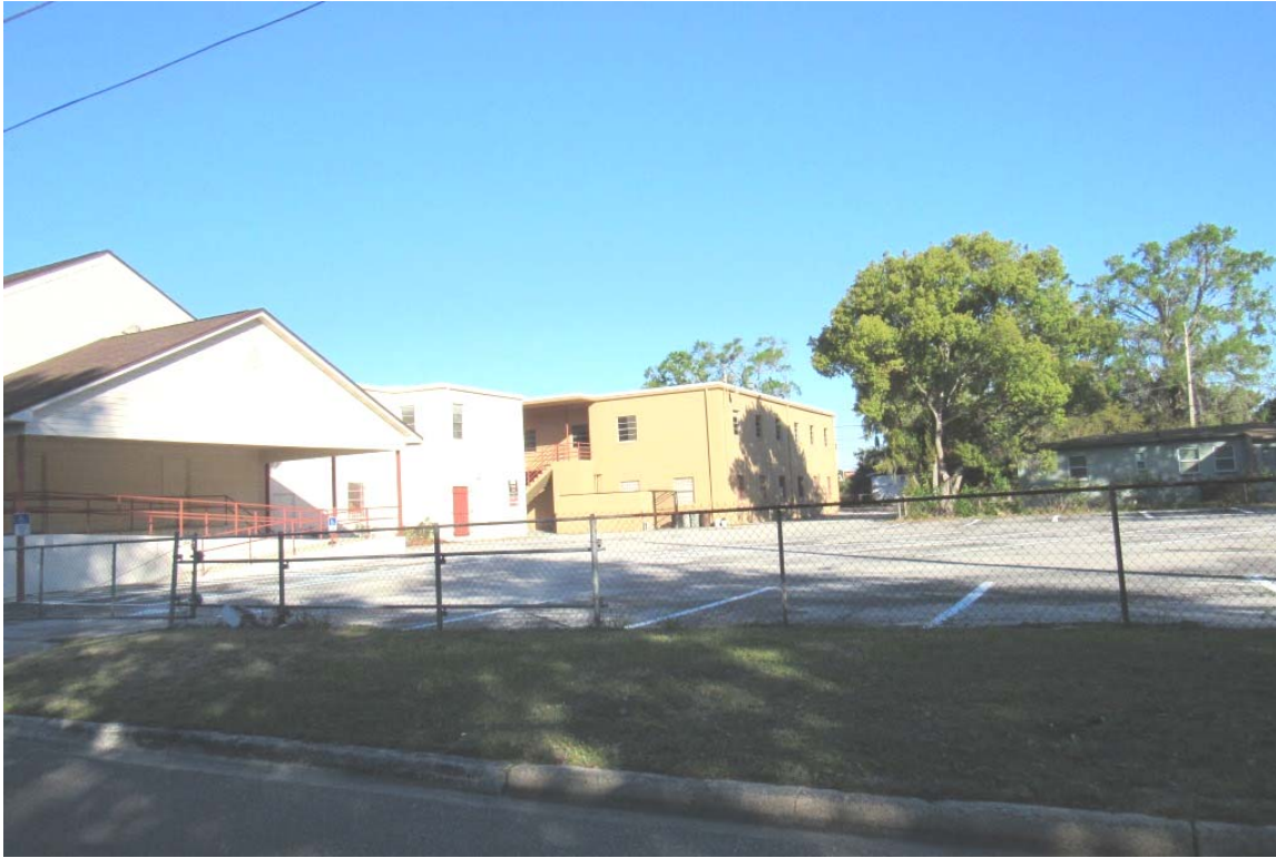
View of parking area from Calvert Street
